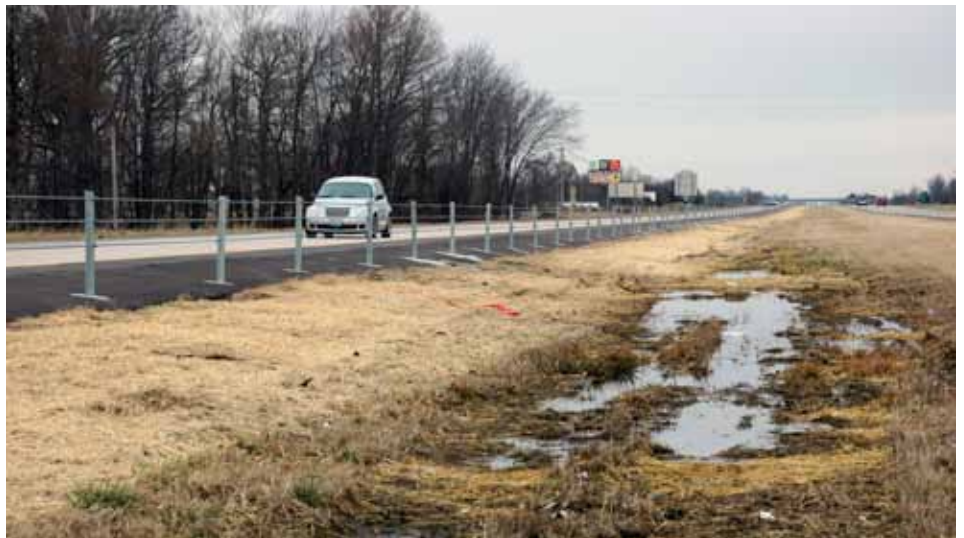
Completed I-55 guard cable system
