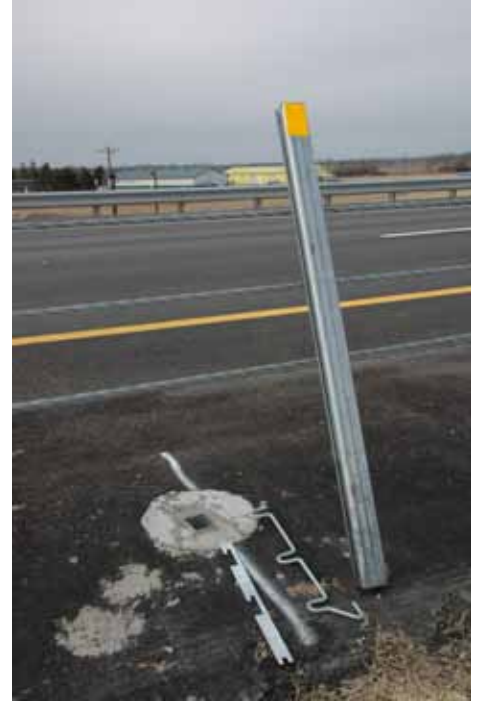
Complete guard cable structure
